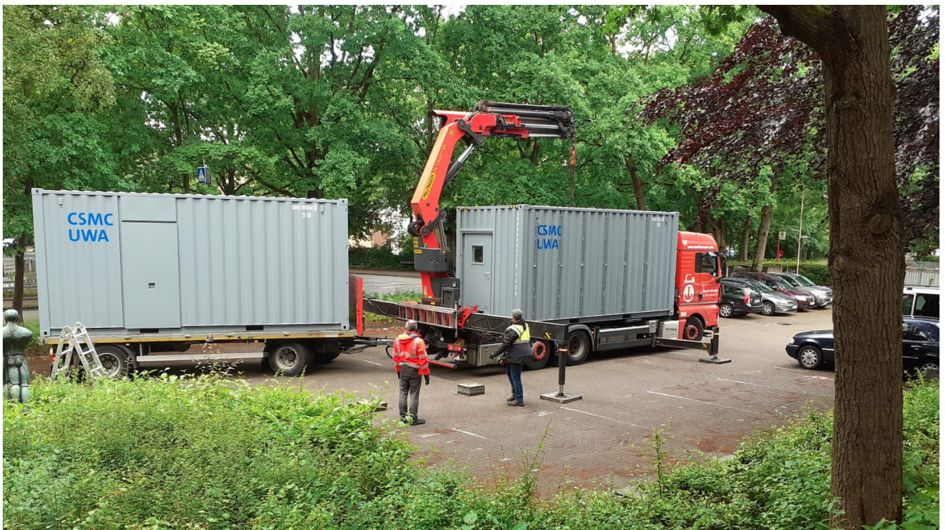
40-tonne crane unloads each container and places it into position
