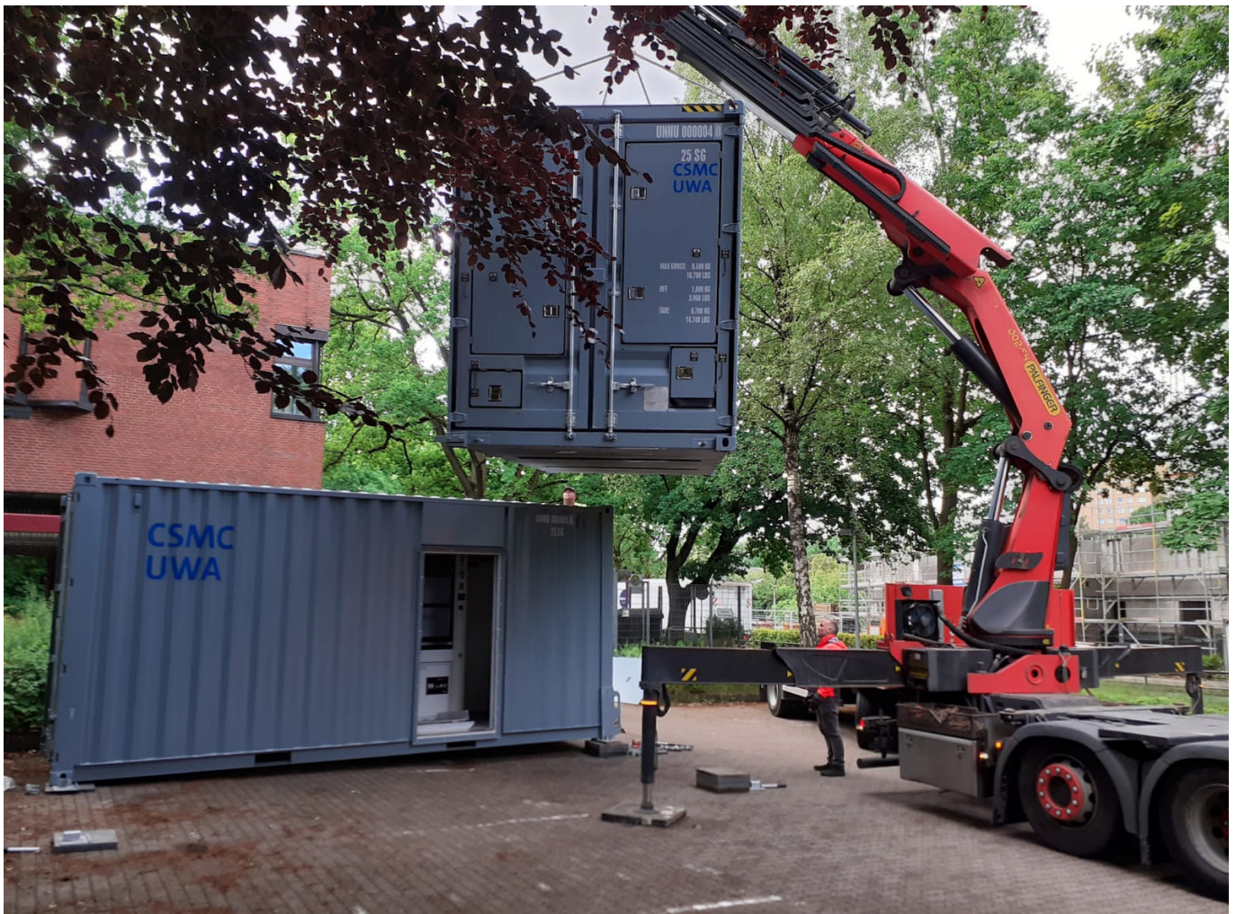
Floor clamps of 8m span provide stability during lifting
